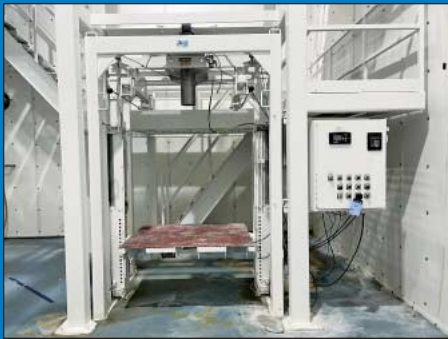
Supersack Bulk Bag Filling and Weigh Station
