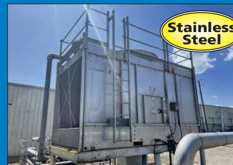
200 Ton Approx. Marley Model NC2211-S.S. Stainless Steel Single Fan Water Tower w/ Pumps
